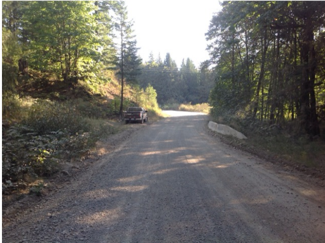
Approach from Right Bank when facing downstream
